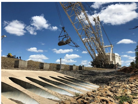
Dragline crossing Smoky Creek to Isaac Plains East
